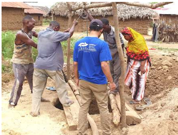
Cutting and fitting of casing pipes
