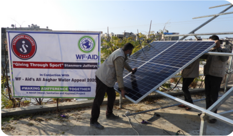
Installation of Solar Panels
