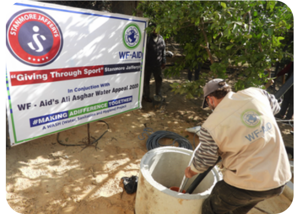
Fitting pipes into the well
