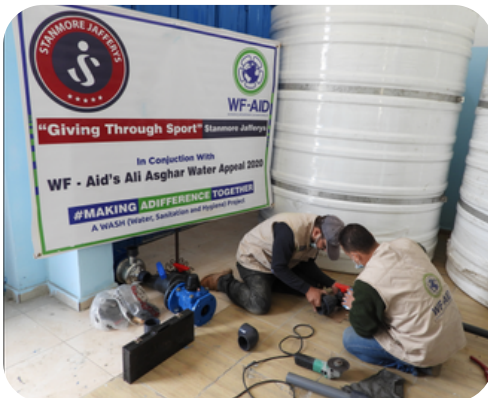
Power system installation
